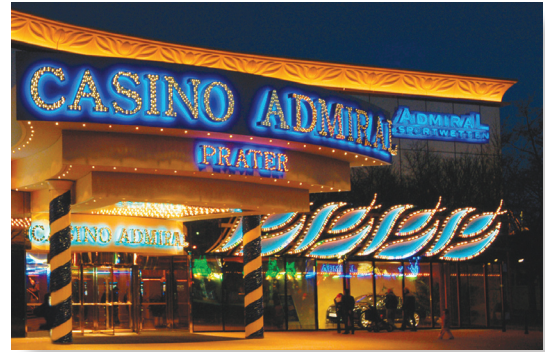
Lightstrings animate channel letters and other features on the exterior of this casino.
